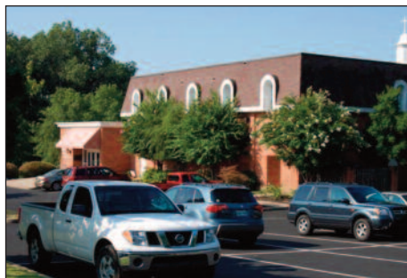
Newly paved parking lot at the OLEC.
